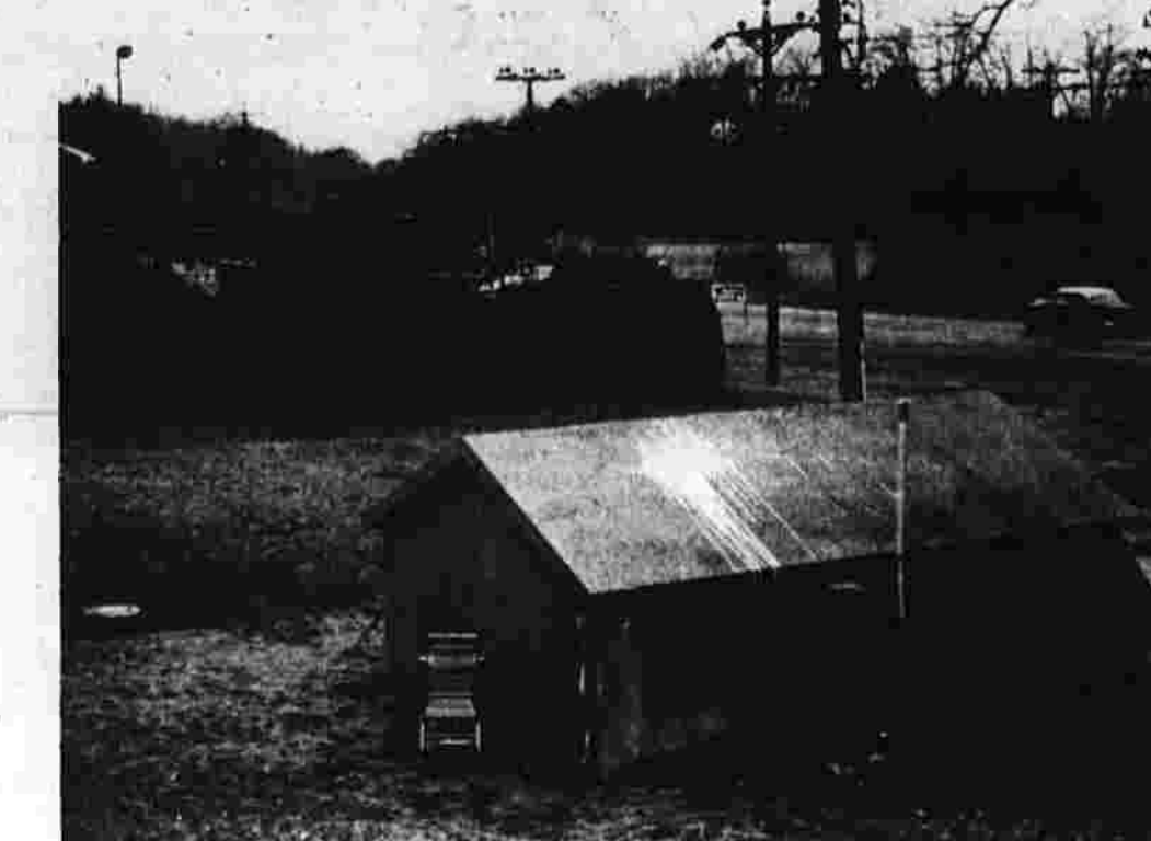
This sewage pumping station is overworked. The result is that Hilliard Pond, in the background, becomes more and more polluted. (Herald photo by Pinto)
